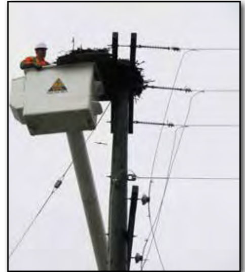
Clayton Olivier, owner of Valley Power Line Contracting, removes the original osprey nest.
